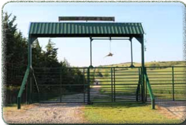
Custom built, electric sliding entrance gate
