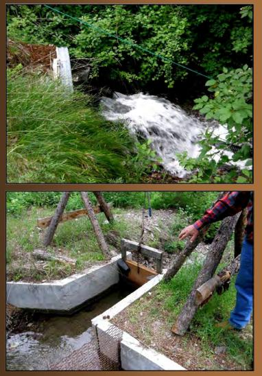
An irrigation and water source starts naturally in the high country and then is directed to Petty Creek. the ranch uses it to drink and bring life to the land. This is engineering at its finest. There's over 5,000 feet in underground piping for irrigating and it is all gravity fed. No pumps! There are sprinklers every 120 feet, giving full fire protection.
